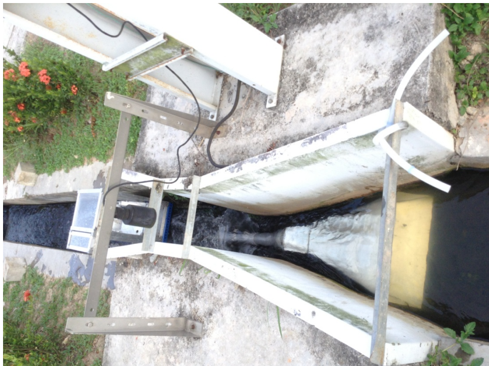
Figure A4: Hydro-system Components in Place at the Drain of Sewage Treatment Plant, UTP
