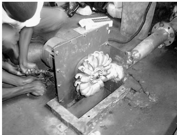
Figure 2.8: Pico-hydro scheme using Pelton Turbine in Kathamba, Kenya
