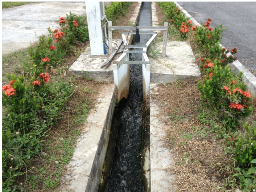
Figure 4.1: The site where measurements are taken for the hydro system project
