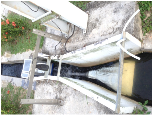
Figure 3.4: Hydropower system at the Sewage Drain
