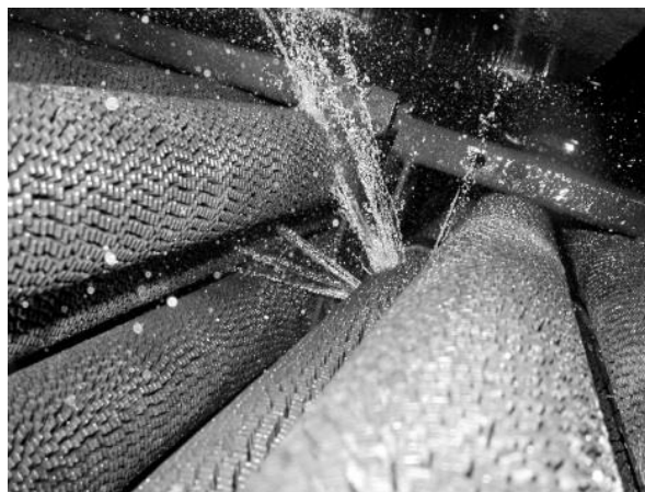
Figure 2.13: Leaking Evaporator Tubes (F.C Anderson, 2003)
