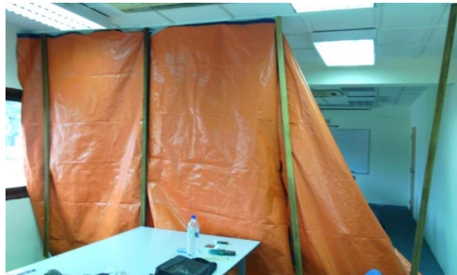
Figure 3.9: Sequential scheme of room's partition construction.
