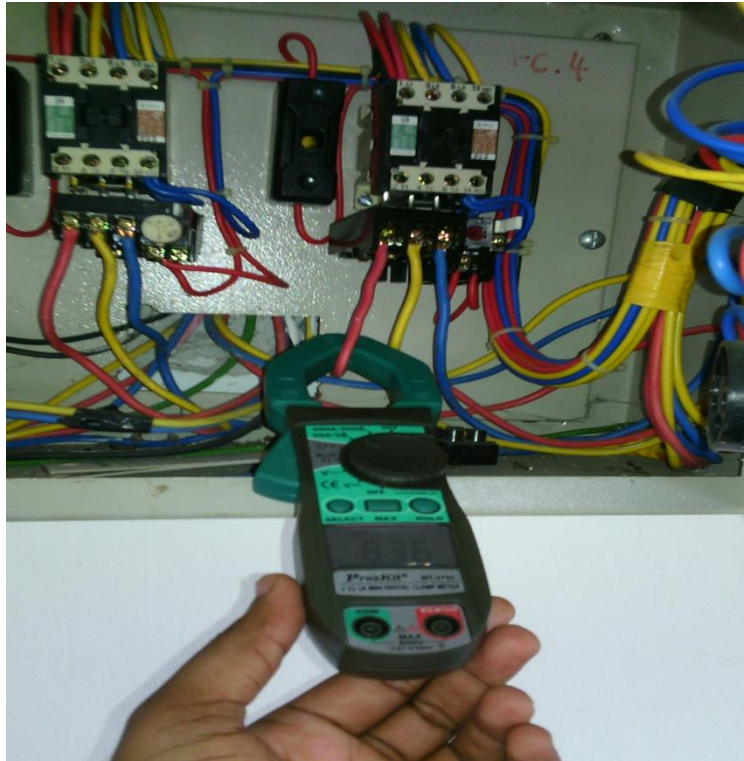
Figure 4.2: Measurement of electrical current and voltage of air conditioning unit using mini multi meter
