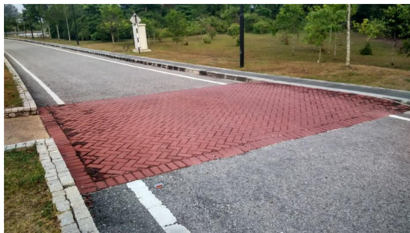
FIGURE 33. Car-Mounted Field testing (Bump)
