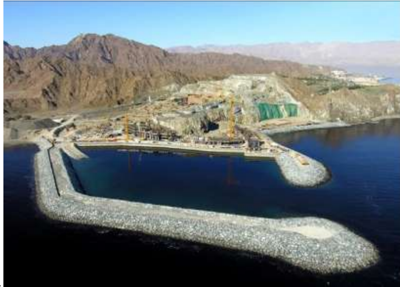
Figure 2 : Breakwater at Mina Al Fajr
