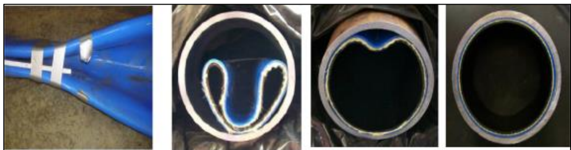
Figure 2.3: IFL installation in a metallic pipe [15].
