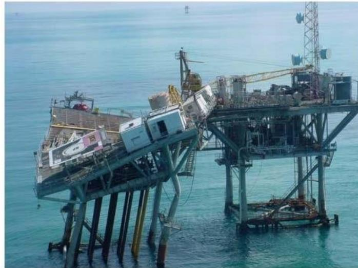
Figure 1.1.1. Two offshore platform damaged during a hurricane off Louisiana
