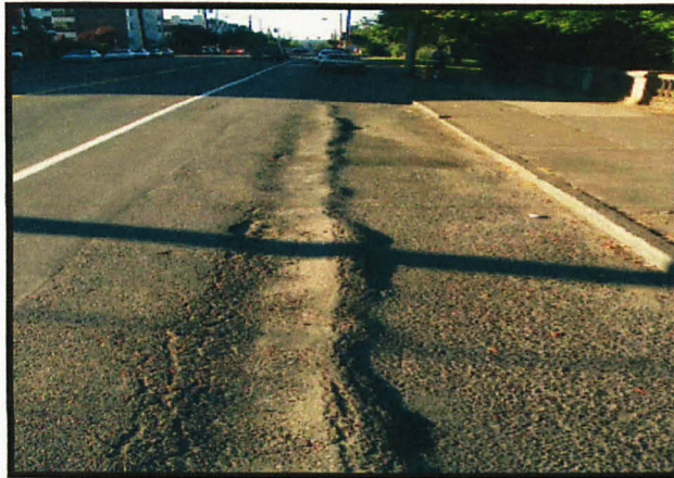
Figure 1: Rutting of pavement structure
