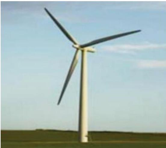
Figure 2.13. Horizontal axis wind turbine.[41]
