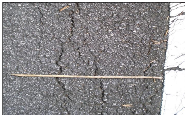
Figure 1-3: Fatigue cracking. (Photo taken from Pangkor. Malaysia, Nov 2008)
