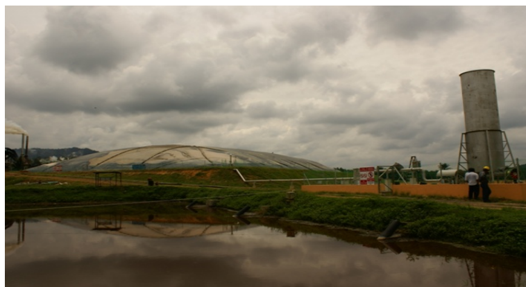
Figure 2.2: Palm Oil Mill Effluent (POME)
