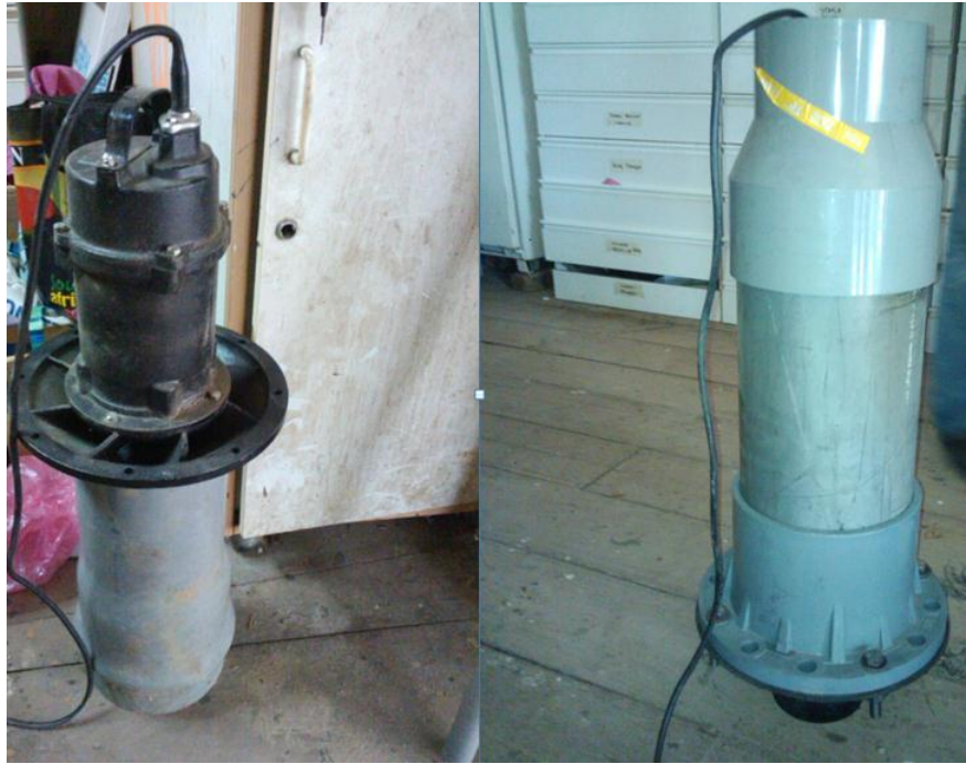
Figure 21: Generator installation in the pipeline
