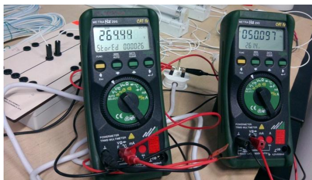
Figure 12: Digital Multimeters monitoring the "No Load" voltage and frequency
