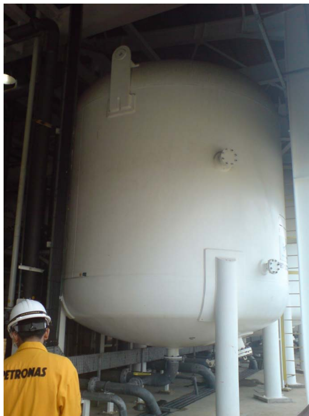
Figure 1.1: Typical Cylindrical Pressure Vessel
