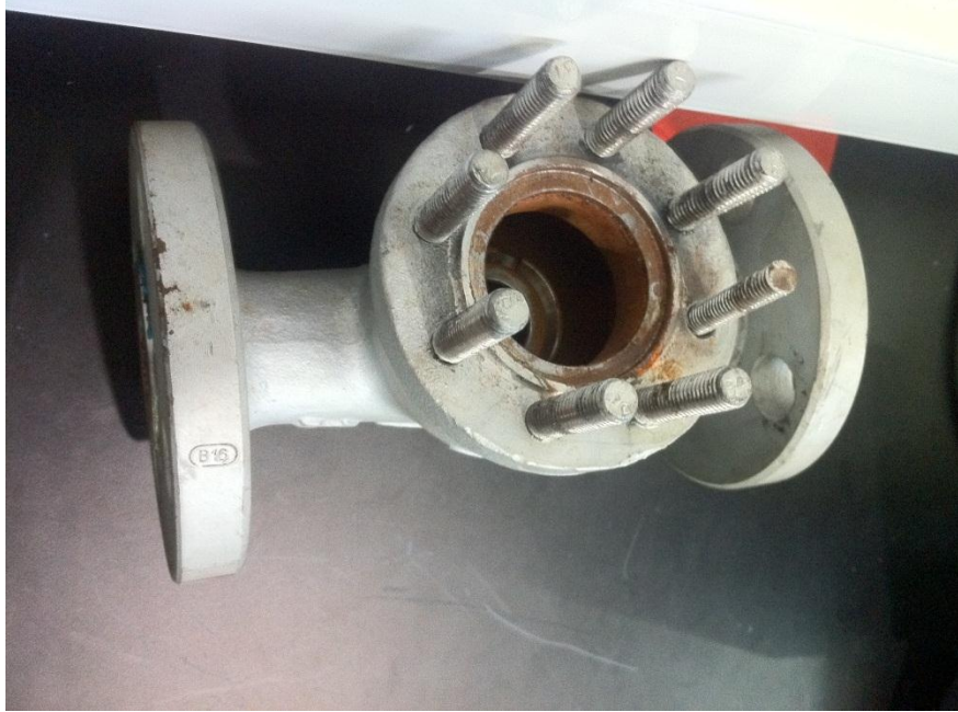
Figure 38 Valve body with a thin corrosion layer
