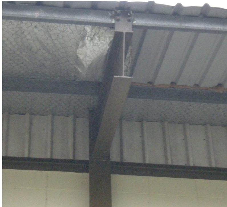
Figure 5: I-beam in structure.
