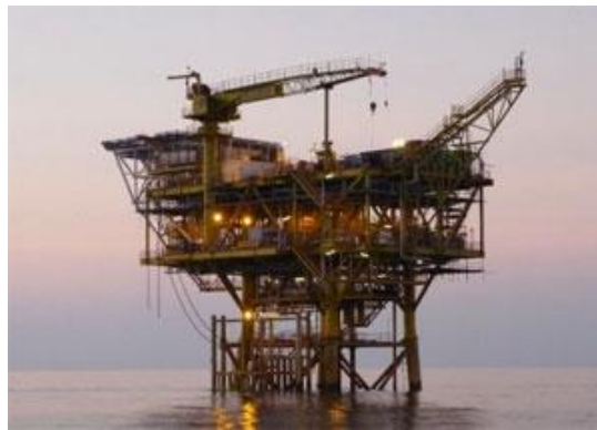
Figure 3: An off-shore steel platform.
