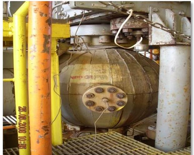
Figure 3 : Spherical Separator
