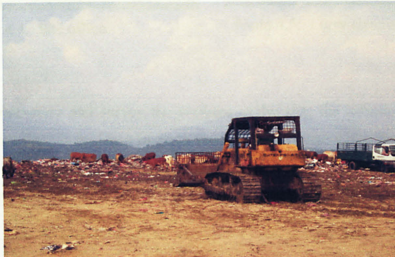
Photo 4.3: Spreading and compacting of waste
