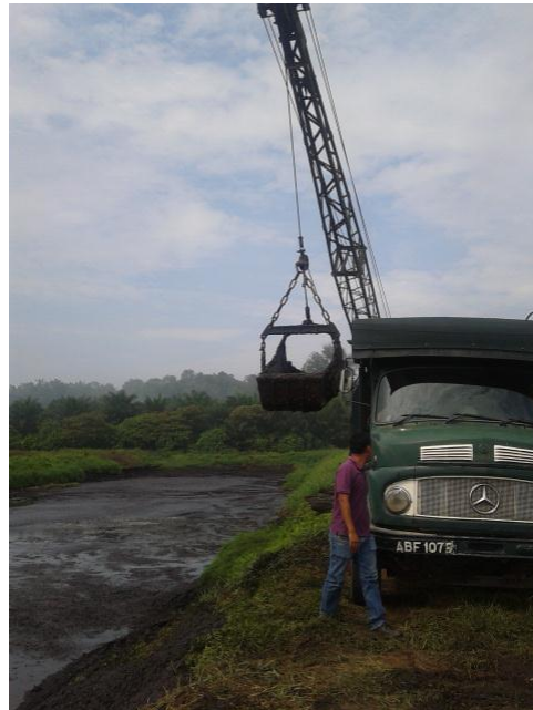
Figure 8.2 Process of Retrieving Sludge In Anaerobic Pond 6, FELCRA Nasaruddin
