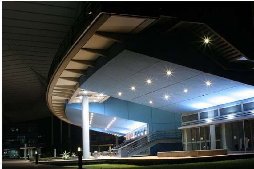
Figure 3.2 Pocket D building
