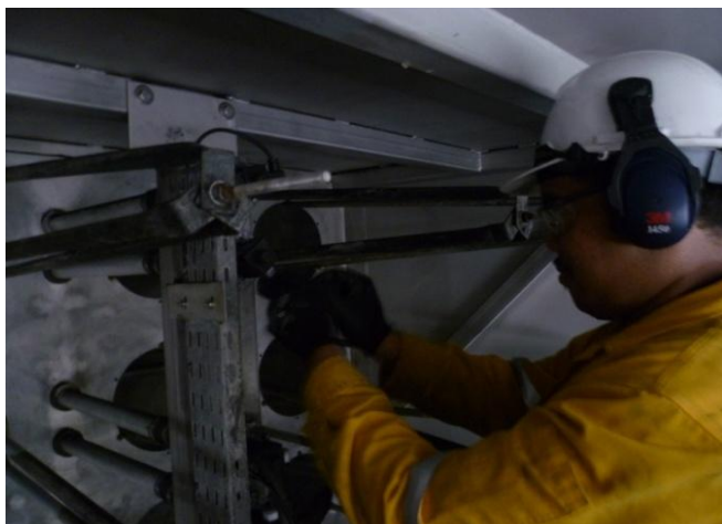
Figure 11: Solenoid valve uninstall work
