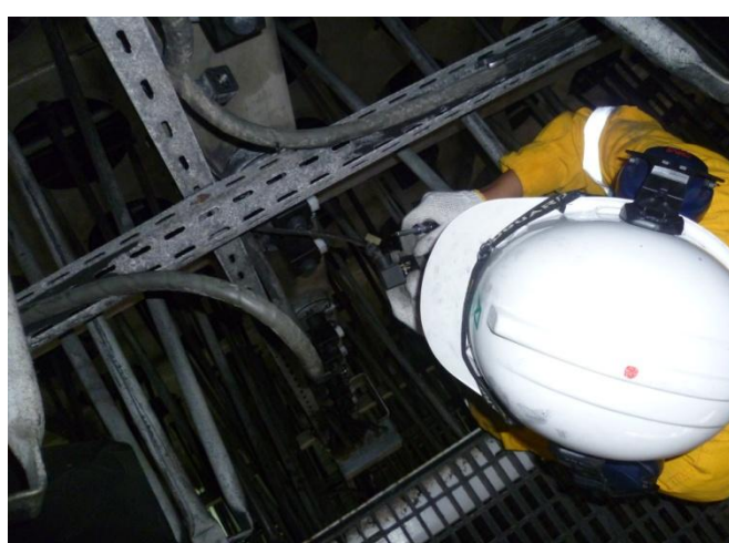
Figure 13: cable socket repairing
