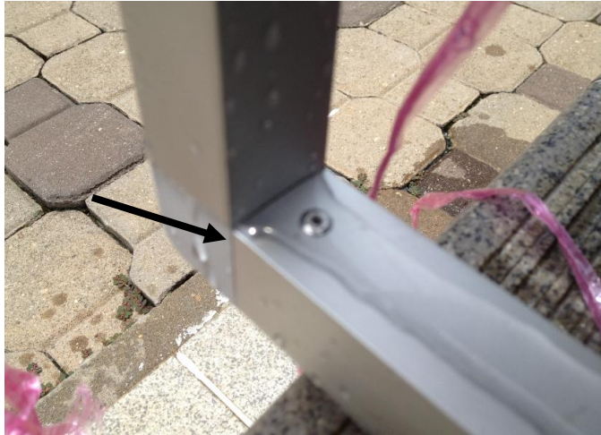
Figure 21 : Leakage at joint
