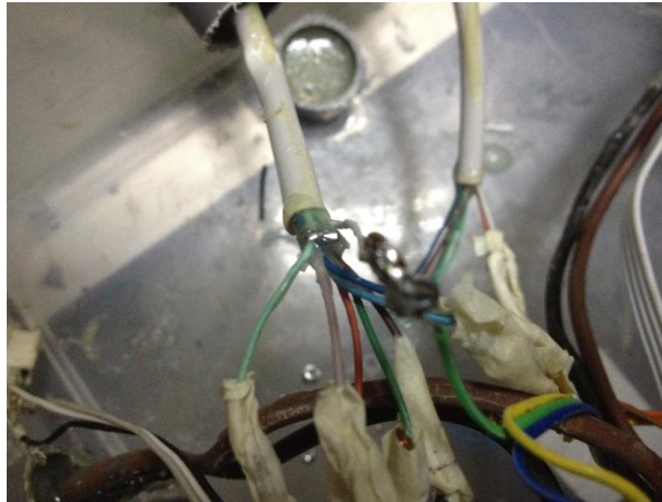
Figure 29 : Epoxy has been applied at the end of the Ethernet cable
