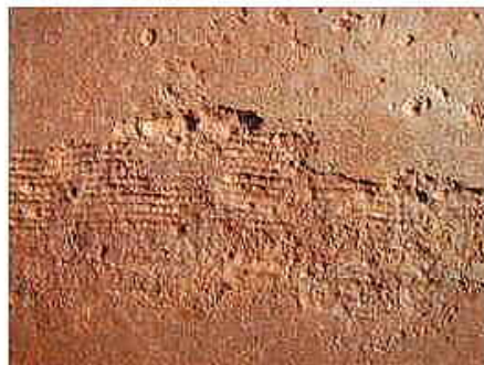
Examples of corrosion striations
