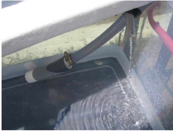
Figure 11: The pump (left side) and TES tank outlet (right side)
