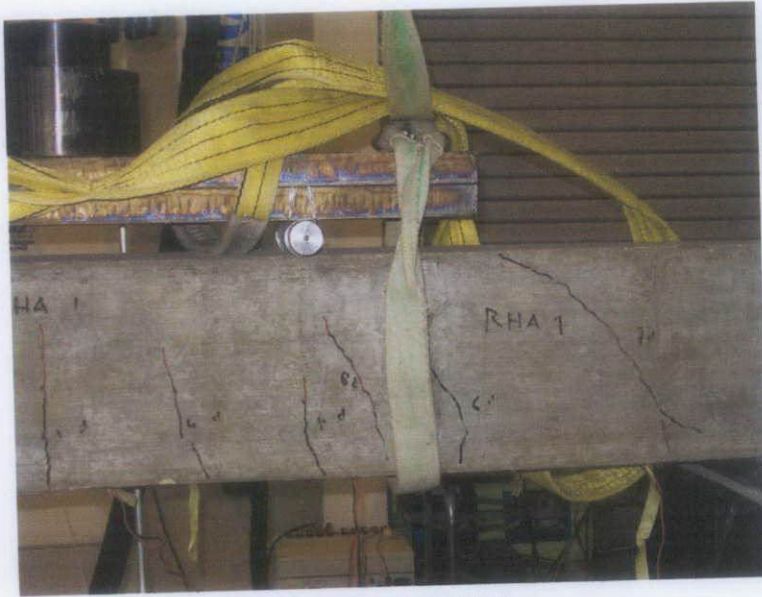
Crack occur at RHA 1
