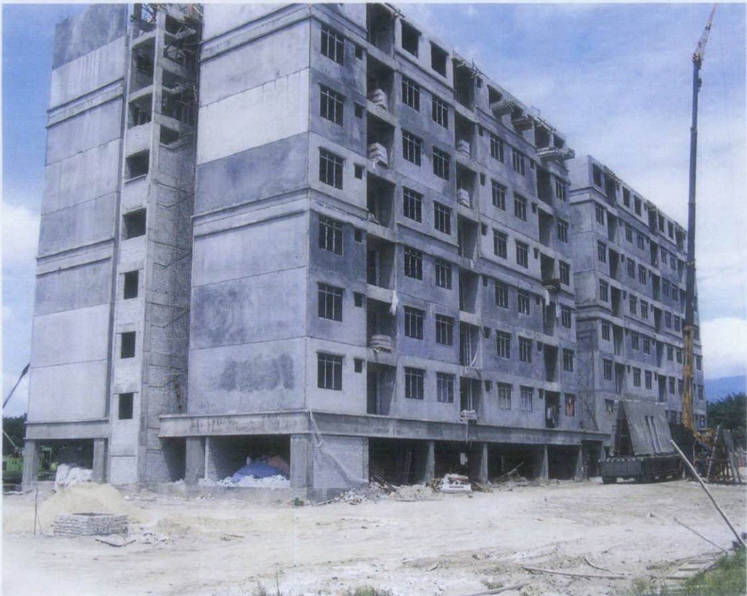
Figure 2.2: Condition of Precast Construction Site
