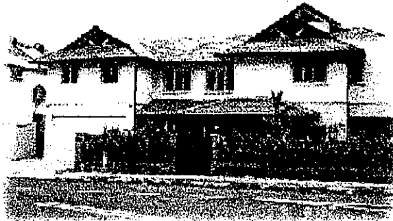
Double storey bungalows in Damansara Heights
