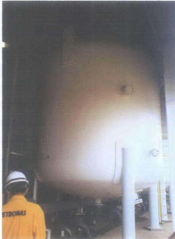
Figure 1.1: Typical Cylindrical Pressure Vessel
