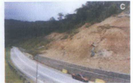
Figure 4.2: Slope at Cameron Highlands
