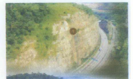
Figure 4.4: Slope at NKVE near Bukit Lanjan Interchange
