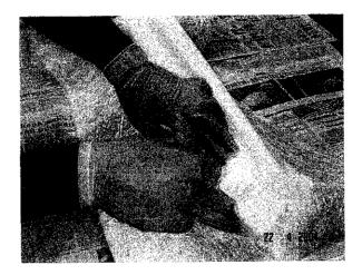
5) Using a roller, polyester is uniformly distributed around the surface
