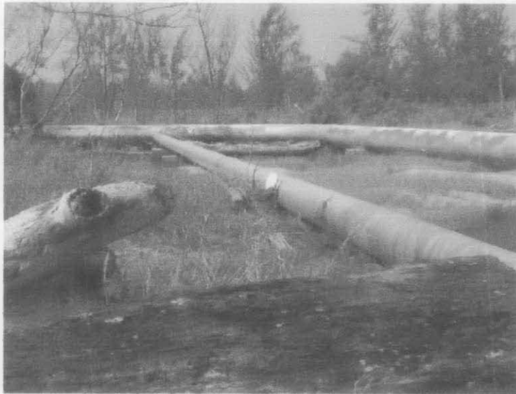
Figure 1.1 Timber logs piling up on pipelines
