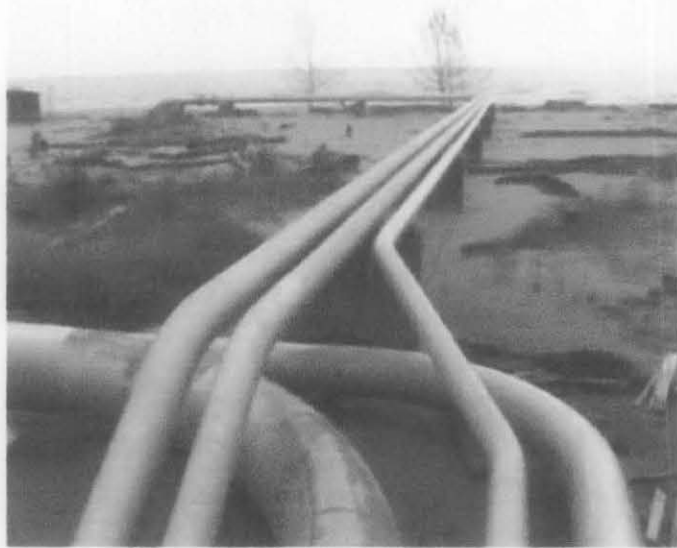
Figure 4.6 Pipelines to be protected
