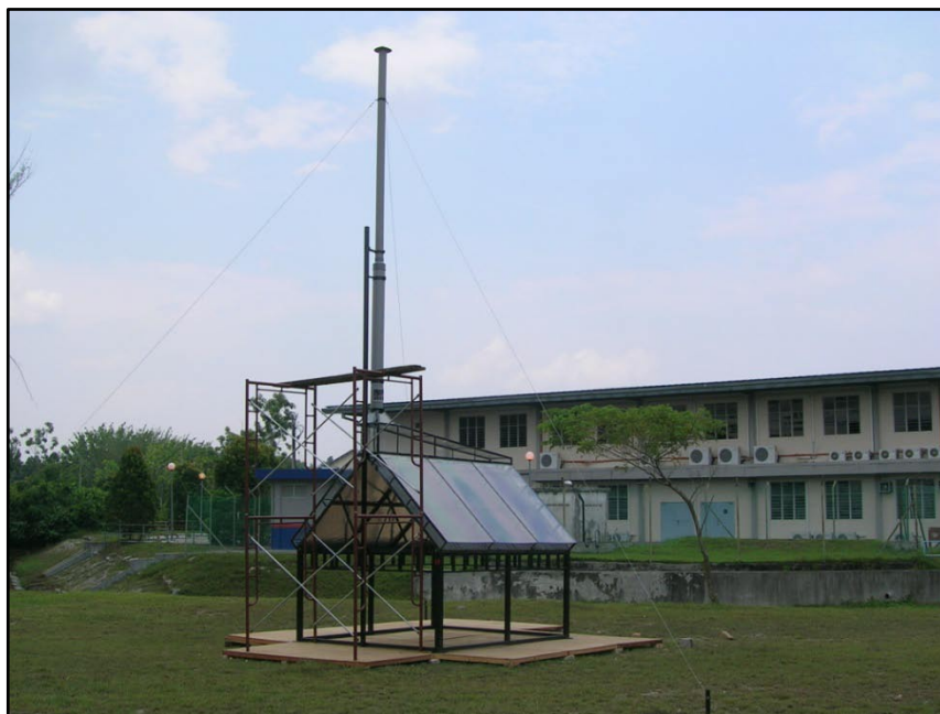
Figure 5.11 Installed and Fabricated on Roof Solar Chimney
