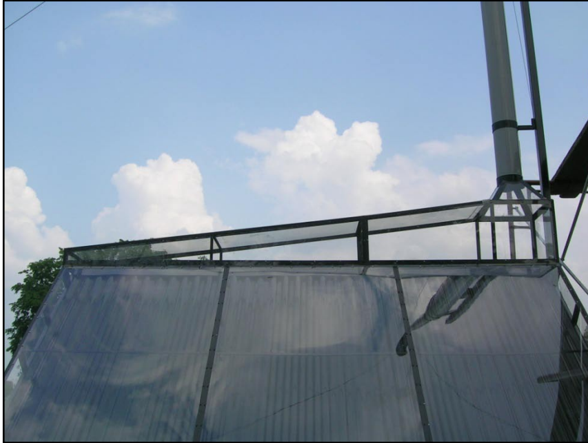
Figure 5.5 Inclined Chimney Cover
