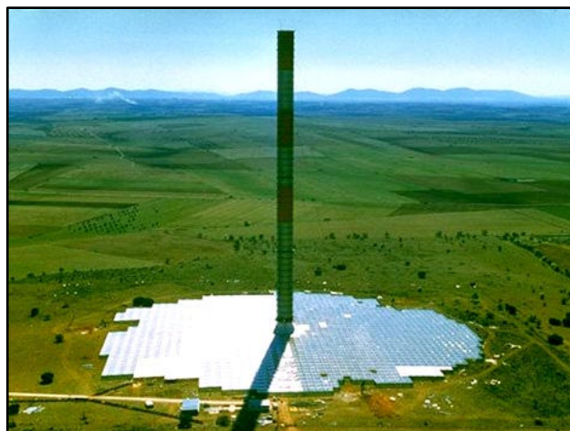
Figure 1.1 Solar Updraft Tower in Spain
