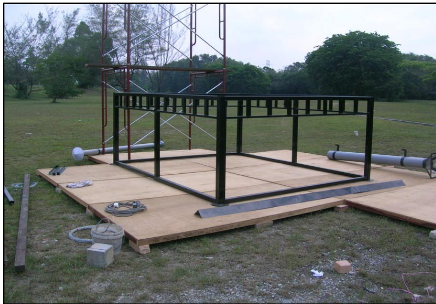
Figure 5.7 The Base and the Structure of the House
