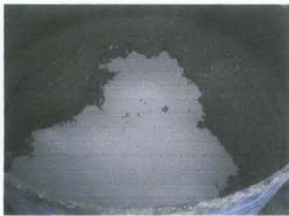
Mixing cement in the mixer
