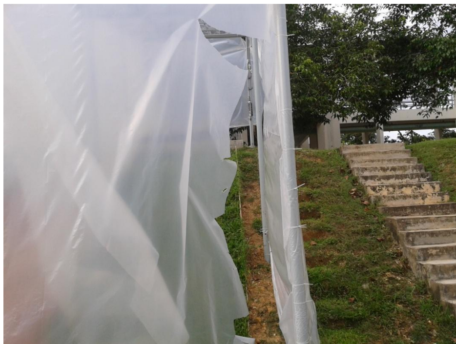
Figure 19: The bottom part has been ripped off due to strong winds
