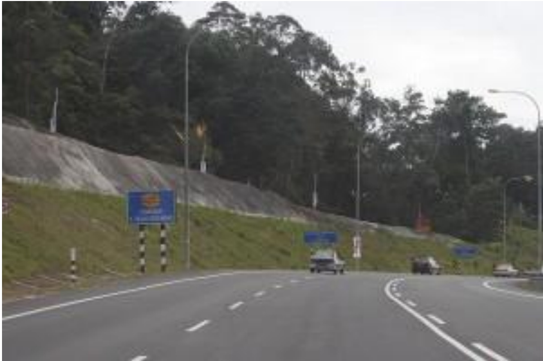
Figure 3: The embankment cover along the highway
