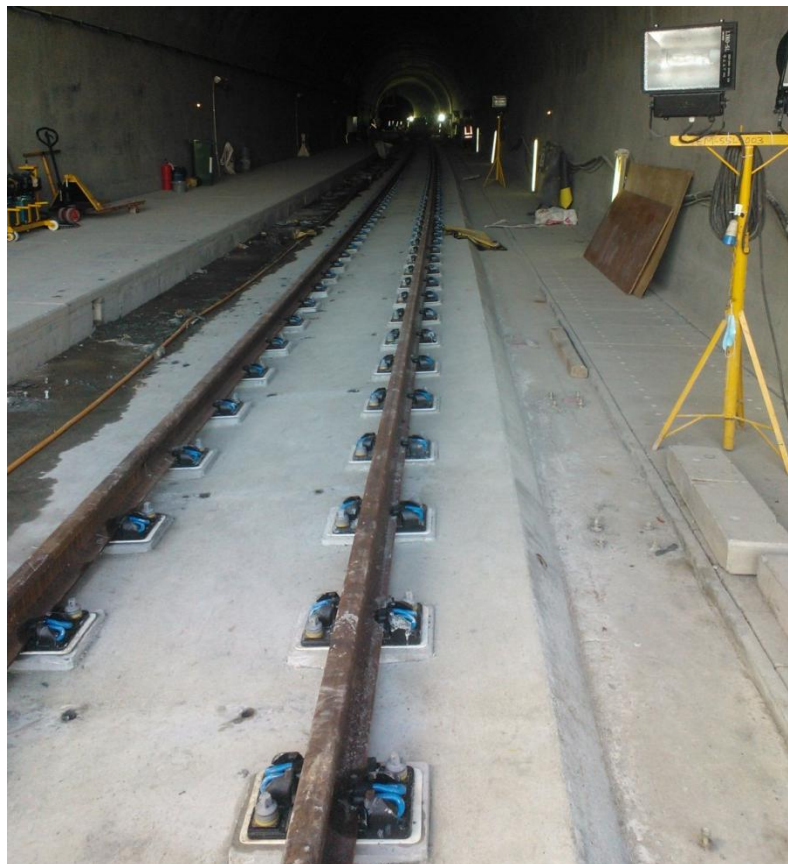
Figure 5: Completion of Concrete Slab Track For Berapit Tunnel
