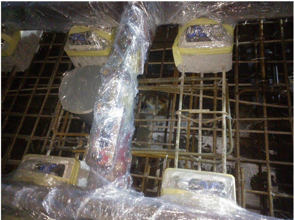
Figure 3: Construction of top slab in Berapit Tunnel
