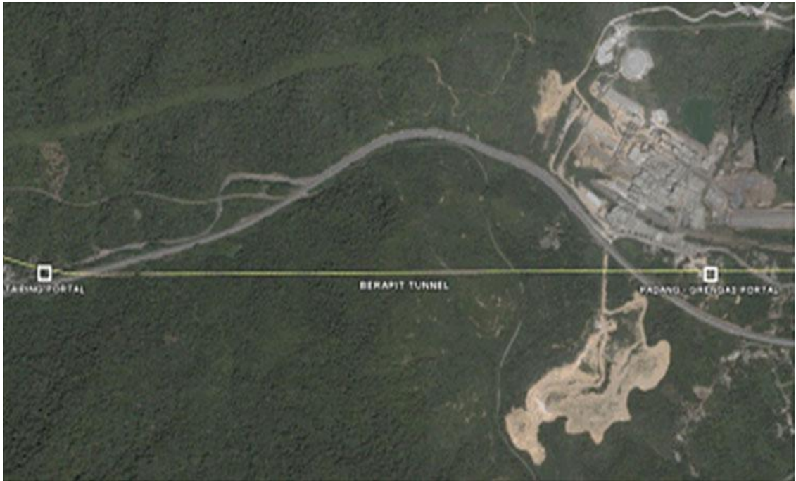
Figure 2: Stretch between Taiping portal and Padang Rengas Portal
