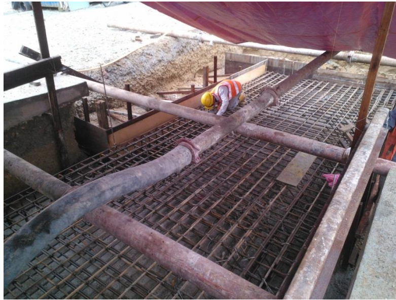
Figure 4: Construction of Transition Slab (excavation work + formwork)
