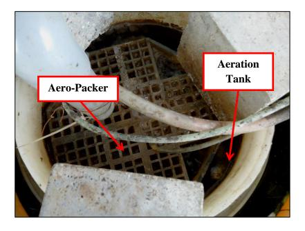
Figure 13: Top View of Aeration Tank after the Installation Aero-Packer
