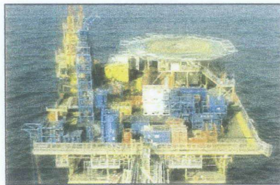
Figure 6: CT Operations on an Offshore Platform [3]
