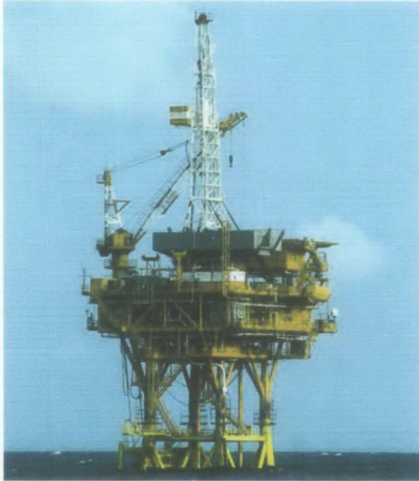
Figure 4: Offshore Workover rig.
