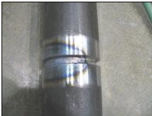
The Heat Affected Zone (HAZ) of a pipe weld, with the blue area being the metal most affected by the heat
