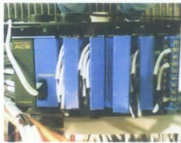
Figure 5: PLC System Chassis
