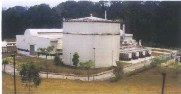
Figure 1: Makhostia Gas District Cooling Plant at UTP
