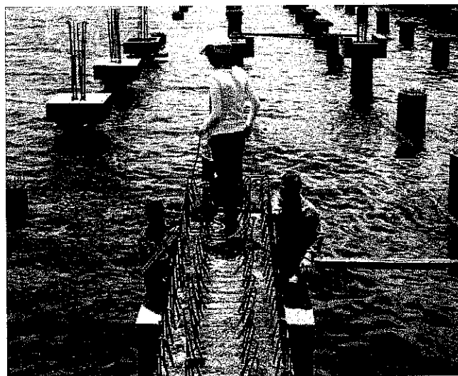
Figure A.2: The first set of frame attached with corrosion coupons (as the control of the experiment) were installed on 24 March 2010 to ensure the dimension of the frames fit the beam.
